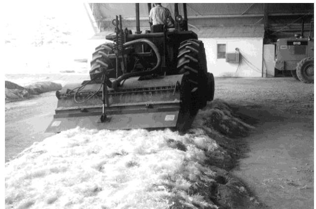
FIG. 7. Mixing Fiber into Sand Using Rotary Mixer
