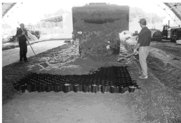
FIG. 8. Installing Sand-Fiber Mixture into Sand-Grid
